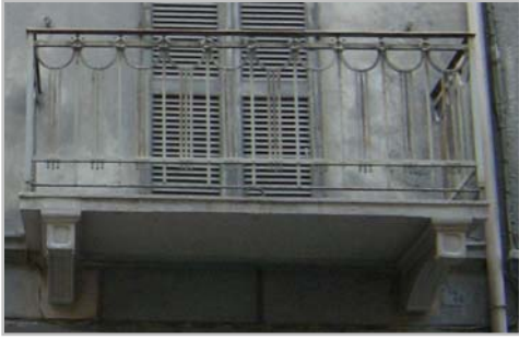
Balcone in cls e ringhiere in ferro
